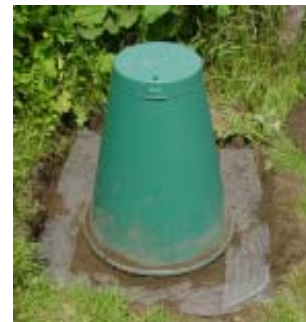
step 6. Hardware cloth placed around the cone.
