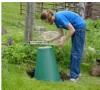
steps 3 & 4. Make sure the rim of the cone is not placed above or too far below the soil surface, and that the cone is level.
